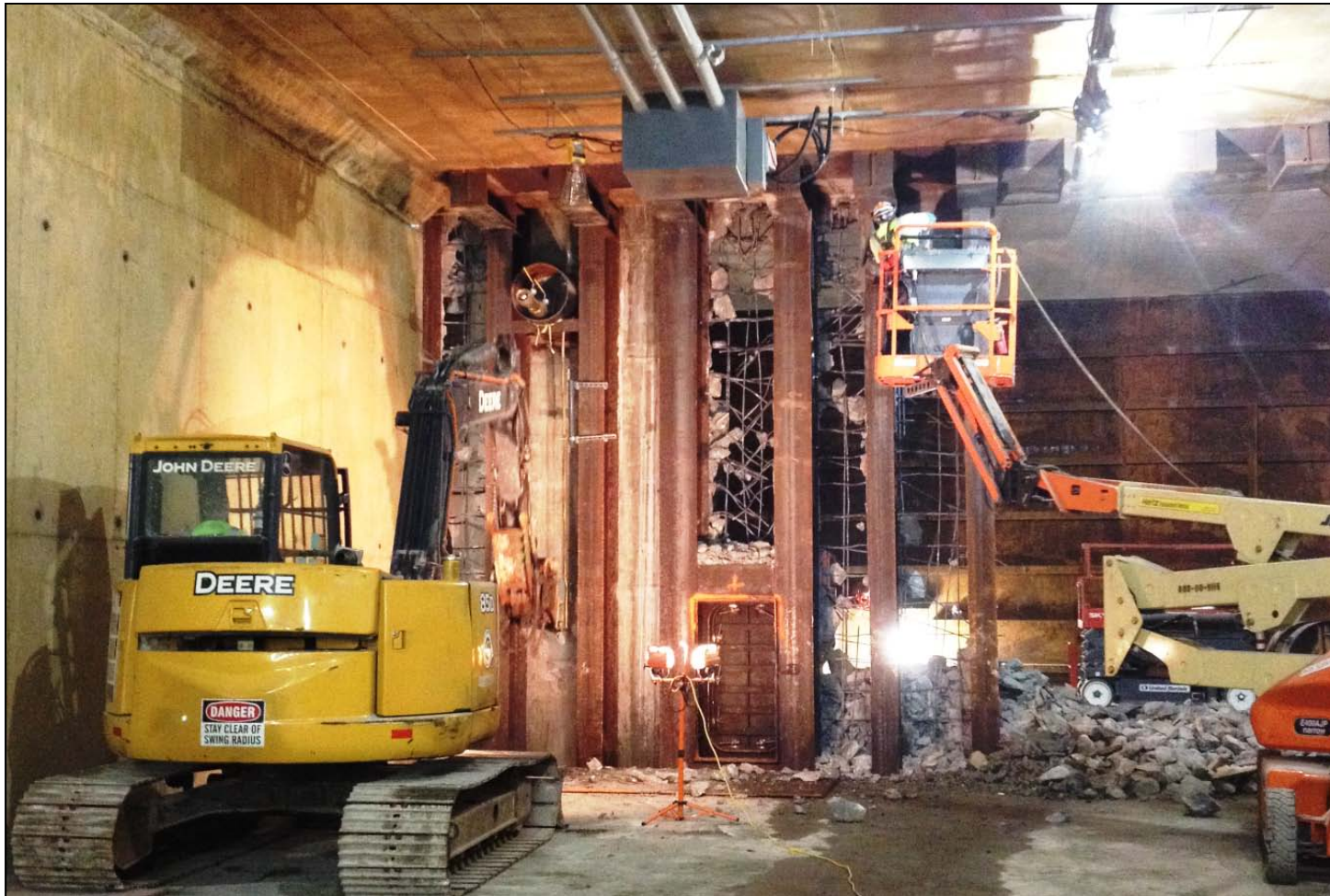
Demo of Temporary Bulkhead N-11 in New MTT (Oct 2015)
