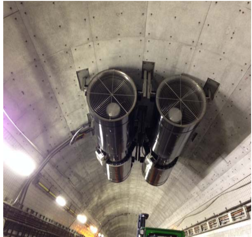
installation of longitudinal ventilation system
