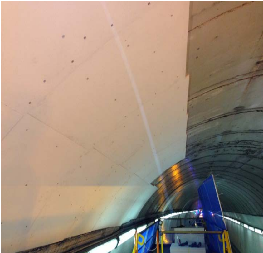
installation of fire protection board
